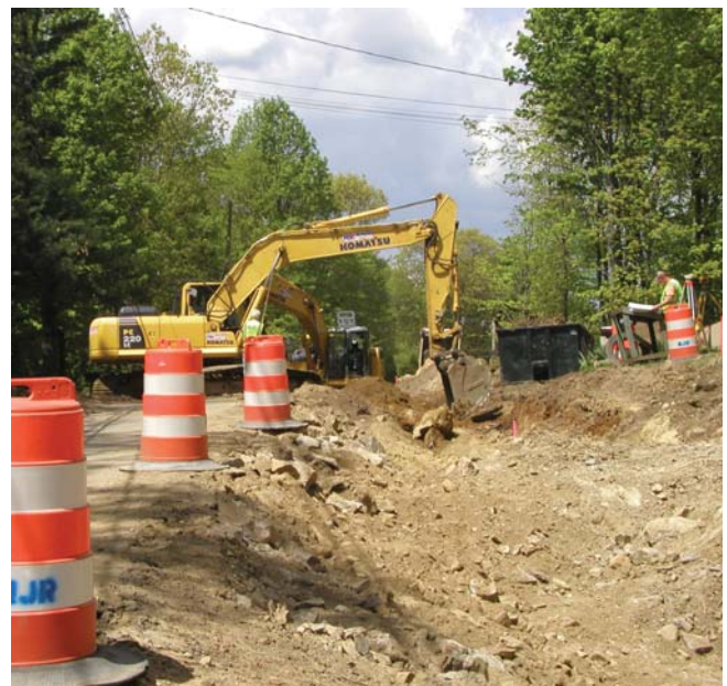
Scott Road Construction, Prospect
